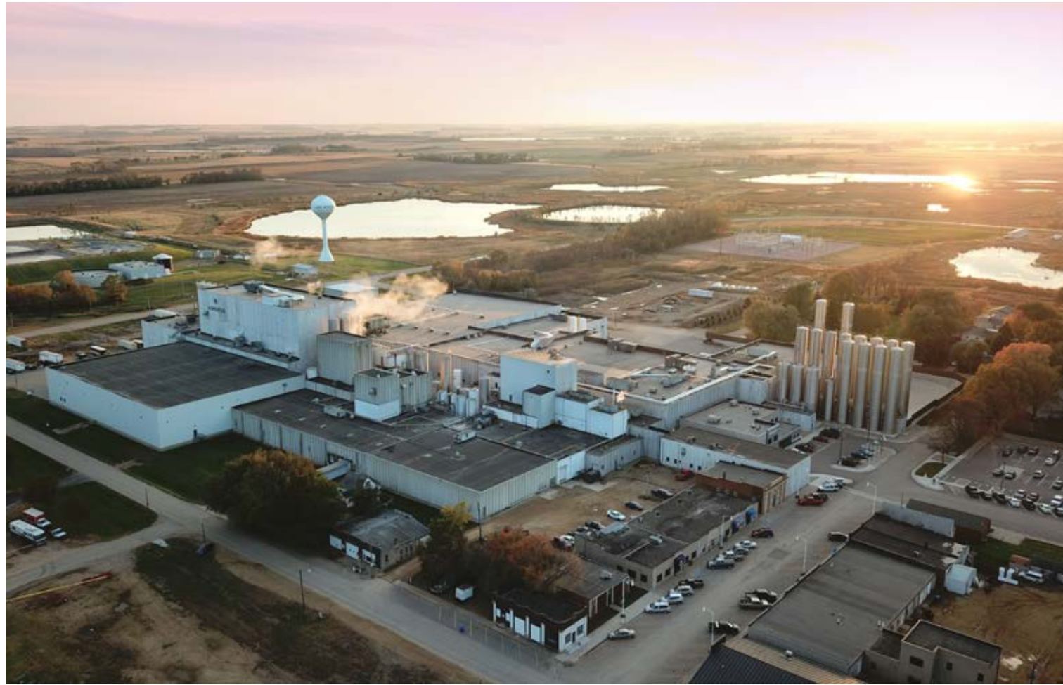
→ The newly expanded Lake Norden plant will be able to make a million pounds of cheese and 540,000 pounds of whey powder daily.
